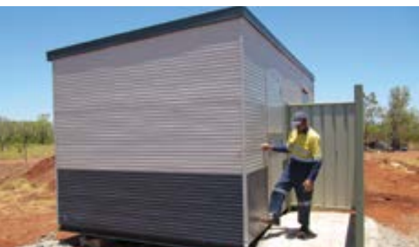
Funding and installing new ablution blocks is one of many ways that GAC maintains and improves the infrastructure in its communities and lore camps
