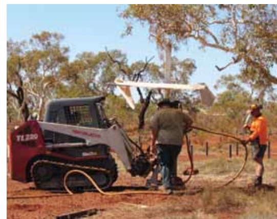
Karijini remediation works in progress
